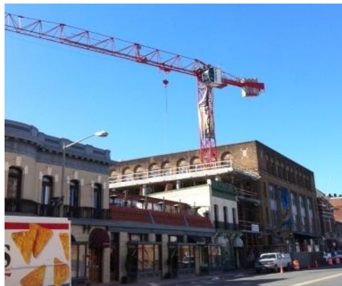
Figure 1: Tower Crane, Picture Courtesy of Luis Ortiz
