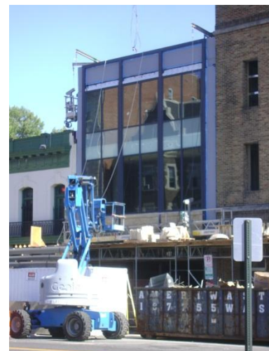
Figure 3: New Addition Curtain Wall, Photo Taken by Clara Watson
