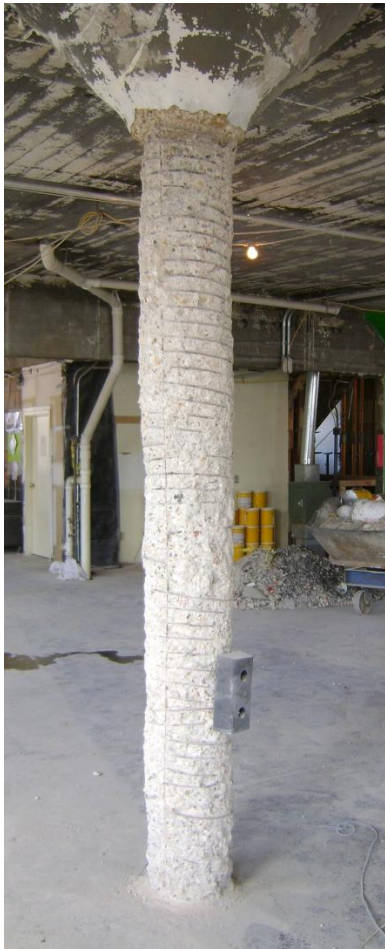
Figure 2: Existing Stripped Column, Courtesy of Luis Ortiz
